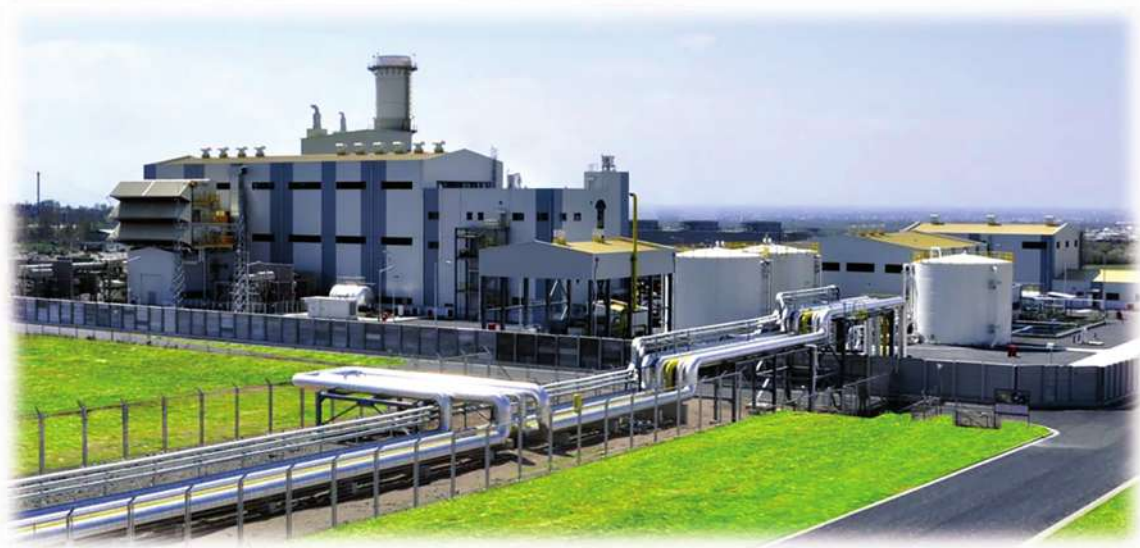
Figure 4. Yerevan Combined Cycle Power Unit, 2010
