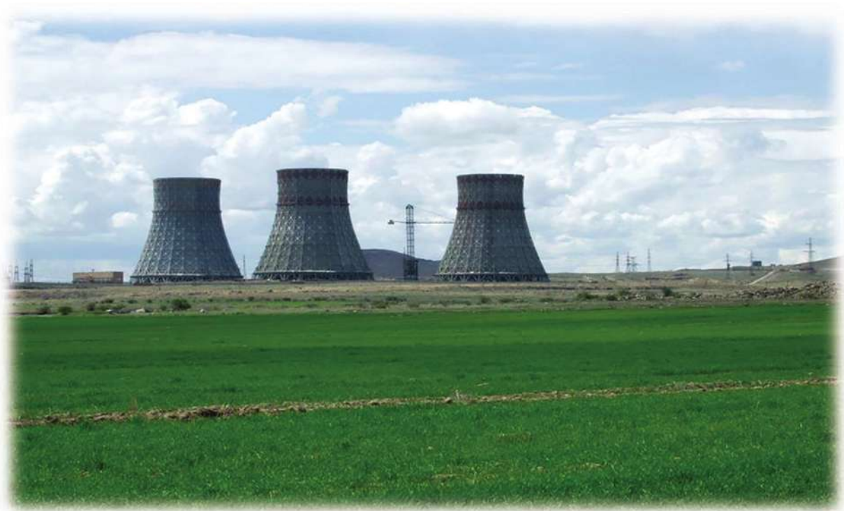
Figure 2. Armenian Nuclear Power Plant in Metsamor
