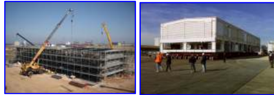
L.E.R., MODULAR BUILDING FABRICATION AND SHIPMENT
