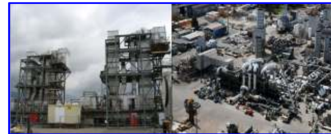
PLANT & PROCESS EQUIPMENT PREFABRICATION / INSTALLATION
